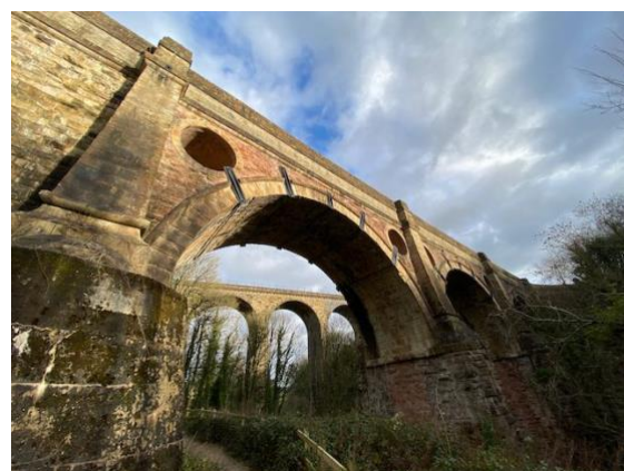
Aqueduct and viaduct viewed from the Goyt Valley
