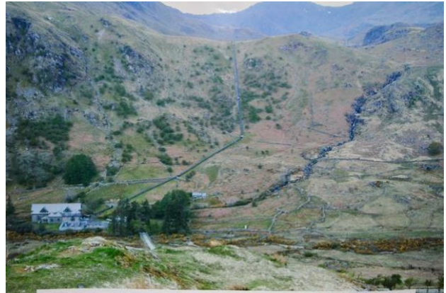
Power station and pipeline from the car park viewing area on the A498 May 2010
