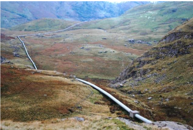
View of completed pipeline restoration October 1998
